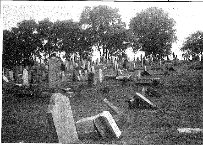
Damage caused by faulty water drainage has undermined the foundations and caused monuments to learn or fall over. The result is a cemetery that looks abandoned or neglected instead of carefully maintained by the community.
